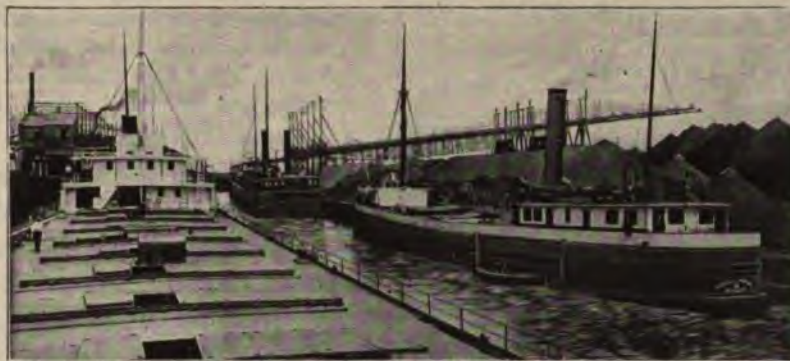
Unloading iron ore from lake steamers at Cleveland. One end of the long steel crane is lowered to the deck; the ore is hoisted and put in cars, which run to the other end of the crane and dump it on the docks.
